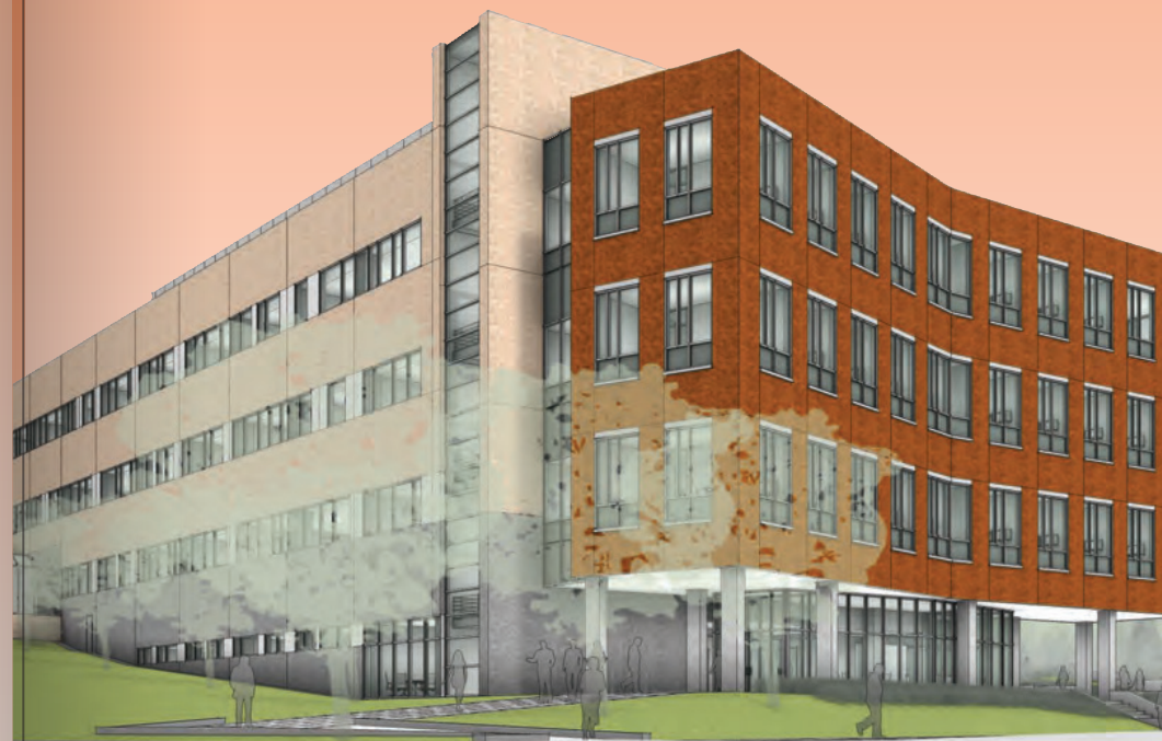
Biology Laboratory Building
